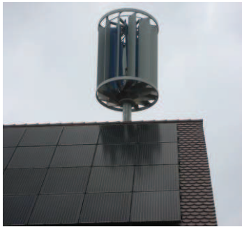
Fig. 1. Installation of a 1kW Turbina VAWT on a rooftop
